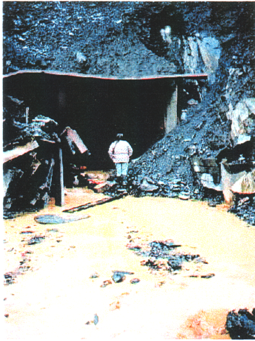
Figure 2 Discharge of adit, September 1998.
